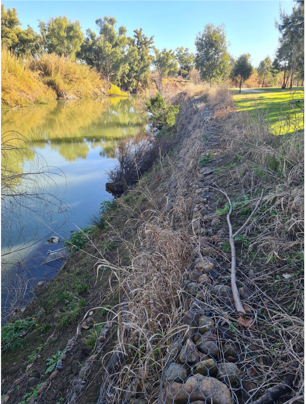
Figure 4: Gabion terracing along northern bank of Peel River to control erosion. No vegetation can establish on this bank.
